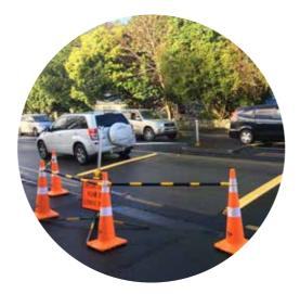
Slowing down the traffic speed with easily adjustable speed humps provides the opportunity to experiment with distances to find the correct spacing to achieve a desired safe speed.
