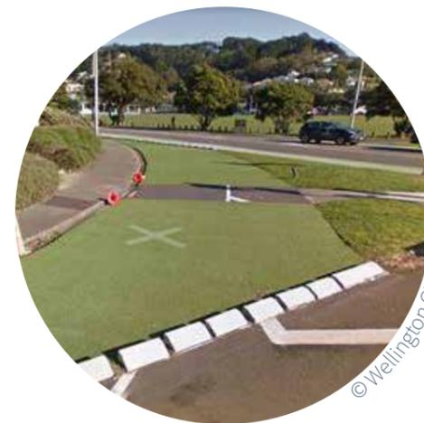
The interim installation allows the impact on the network to be tested over a longer period of time, to monitor changes in behaviour if any.
