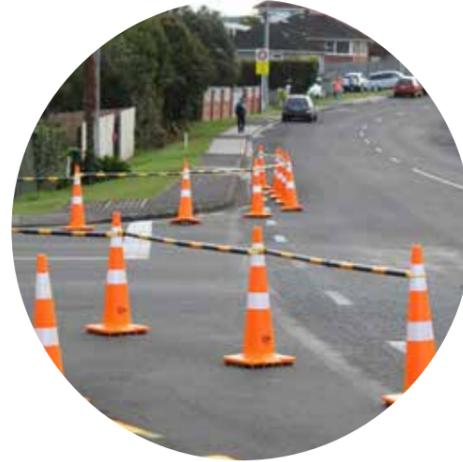
The intersection is tightened to test the maximum space necessary for a turning vehicle, and the impact on conflicts between pedestrians and vehicles.
