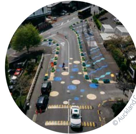
Implementing a temporary crossing at a side road intersection can signal a change in environment from busier, faster arterial roads to slower, local streets. This tool can also provide interim safety and walkability benefits in advance of a permanent upgrade.
