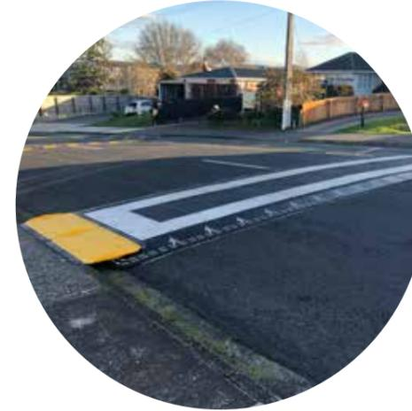
Durable, semi-permanent speed humps or table installations allow time for drivers to adapt to new conditions, and can be altered if required.
